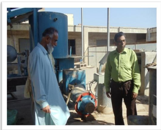
Figure 13. Pellet mill is working to produce pellets for lightweight aggregate
