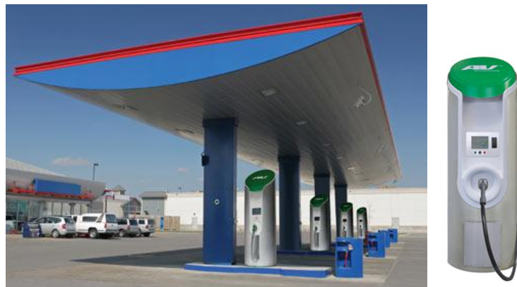
Fig 6. A modern electric Vehicle rapid charging station
